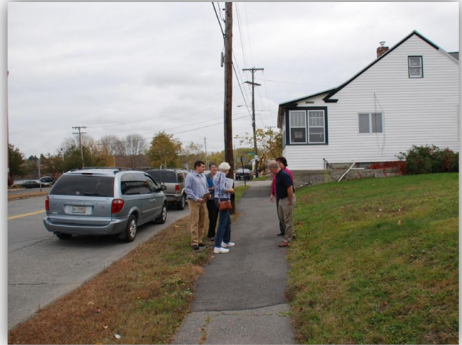
Most of the Downtown Sidewalks have Hot Mix Asphalt Surfaces with either Granite or Bituminous Curb, However Some Sidewalk Surfaces are Concrete and/or Brick.
