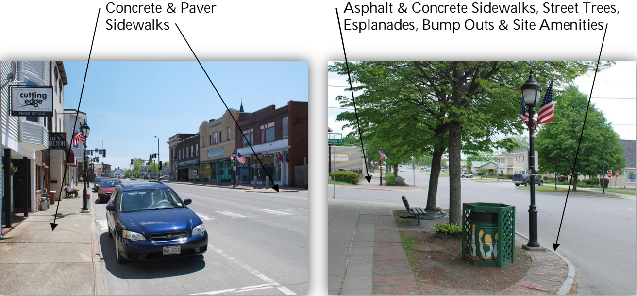
Variety of Considerate, yet Inconsistent Sidewalk and Streetscape Materials on Main Street
