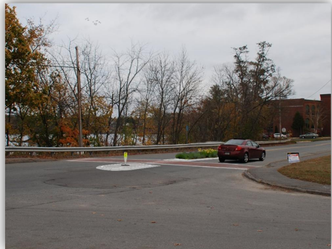
Example Rendering of Raised Median and Year Round Crosswalk Demarcation at Brunswick St and Main St Intersection
