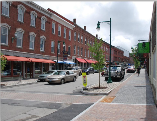
Example of Bump Outs, Concrete Paver Crosswalks and Sidewalks, and ADA Detectable Warning Devices from Downtown Rockland
