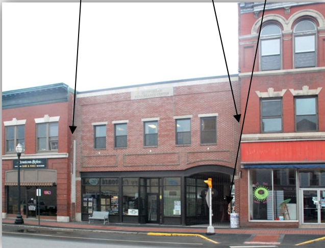
Example of Shared Elevator Access and Second Floor Through Connection in Downtown Skowhegan
